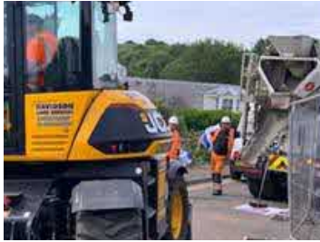
Gabions being installed adjacent to proposed development site
