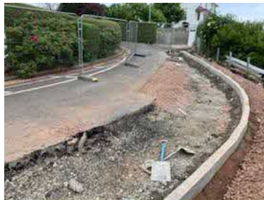
Road being prepared for re tarmacing
