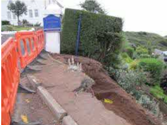
Blue metal sign post and the hedge at acute angles leaning downwards to the coastal slope
